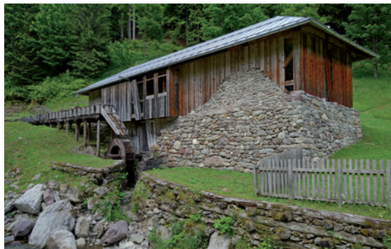
Figure 6 – Valcanza sawmill (1,200 m), reconstructed by Parcopan. © Oliver Bender
